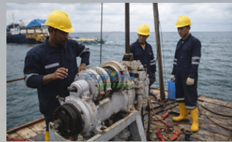
Soil Investigation in Sambu
